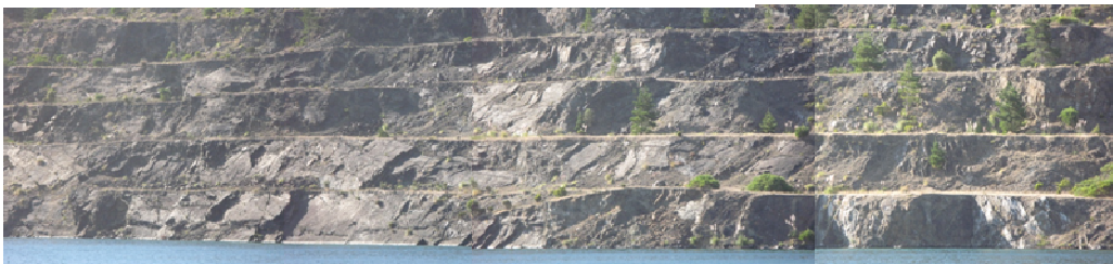
Figure 11 The north wall of the existing open pit viewed from the southern side of the pit. Most batters on this wall are controlled by the dip of planar to undulating geological structures.
